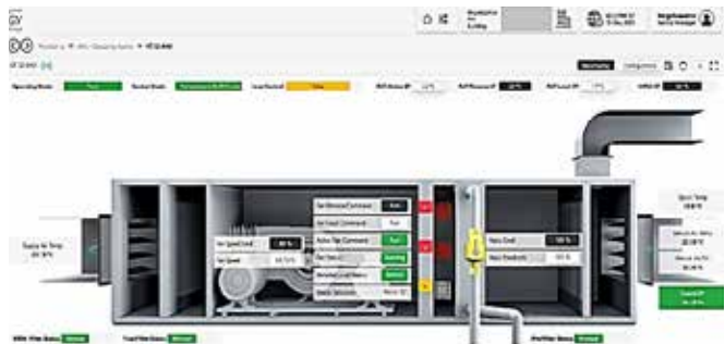
Figure 3: Cloud-based Monitoring and Control dashboard for an AHU
